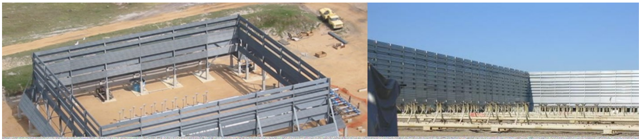
Figure 1 – General Multi-Point Ground Flare (MPGF) with tips and wind fence design
