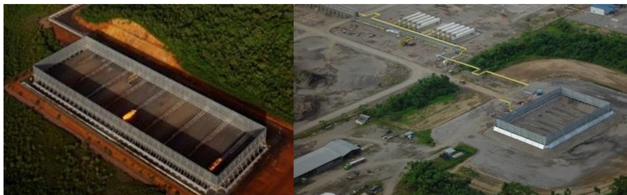
Figure 2 –MPGF are generally located away from main plant to prevent damage to surround equipment
